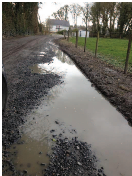
Figure 17: walkway showing poor maintenance
