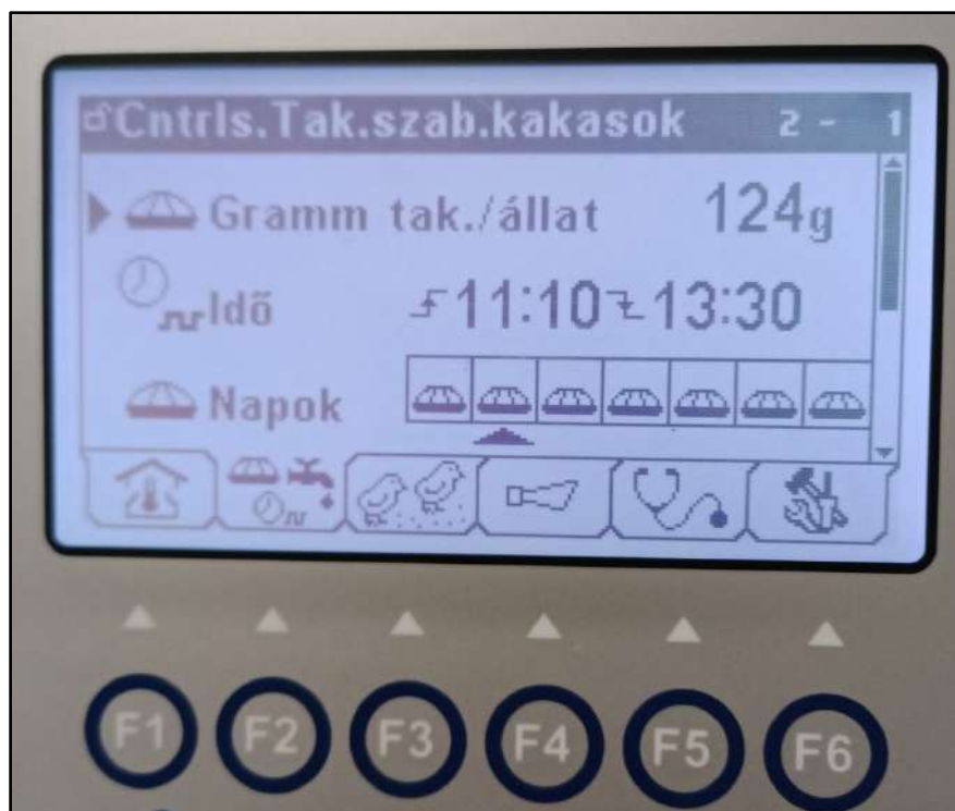
Figure 12 (above) The control panel for the barn located near the barn entrance. Here control over the weight of feed, water and light programs can be made. This particular screen is for altering the feeding settings.
