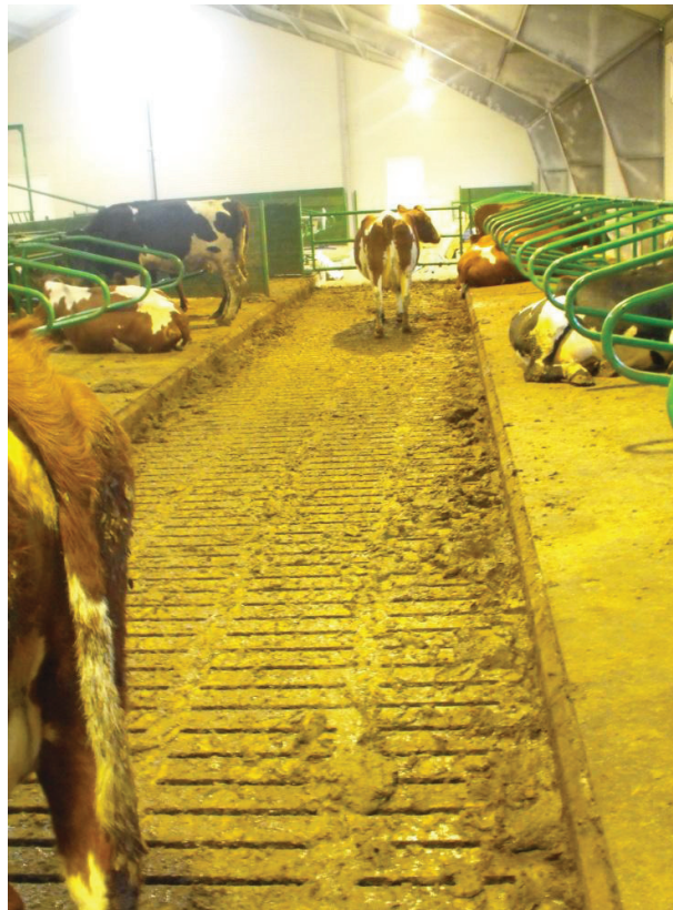
Figure 6. Buildup of faces by the cubicles due to no scraping.
